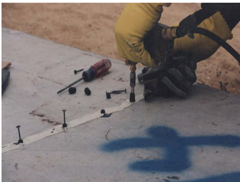
Figure 12. Automatic metering, mixing and dispensing device used in a <math><1/16</math>-inch crack slab specimen [21]
