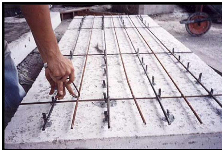
Figure 8. Roughened surface and steel provided and prepared for casting the extra 5cm layer of concrete [2,4]
