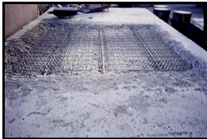
Figure 5. Wired mesh used for repair [2]
