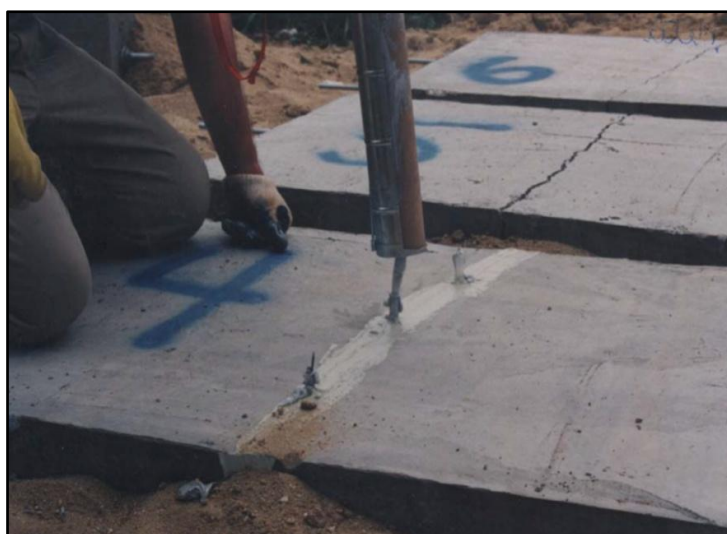
Figure 13. Caulk gun used to manually dispense the epoxy mixture in a 1/4-inch crack slab specimen [21]
