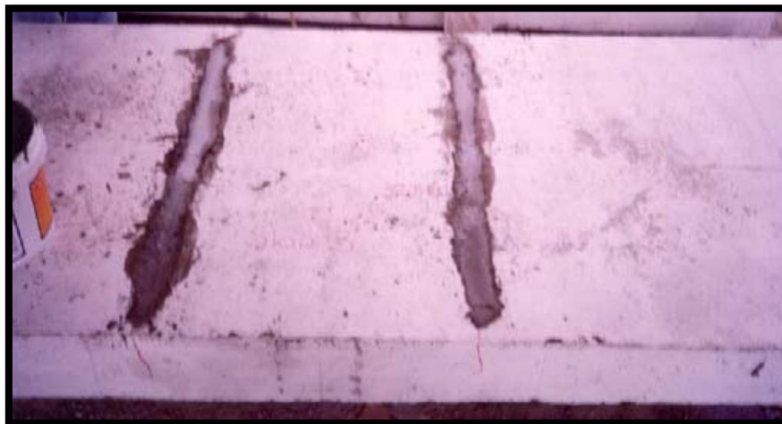
Figure 7. Cracks repaired using grout pouring technique [4]
