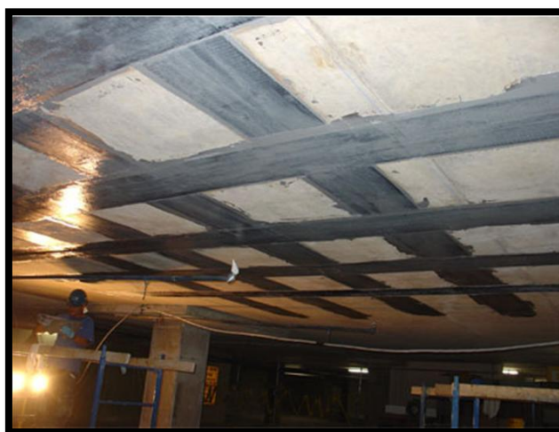
Figure 1. Strengthening and repair of bridges using CRFP laminates [8]
