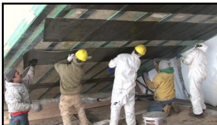
Figure 2. Strengthening and repair of bridges using CRFP laminates [8]
