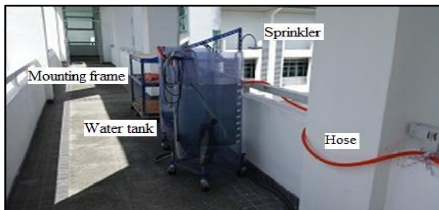
Figure 1: Sprinkler is attached to a steel frame to stabilize flow of water.
