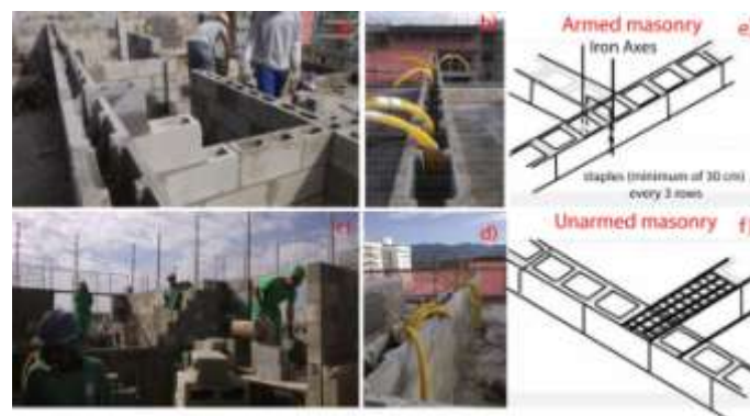
Figure 5. a) First elevation of masonry, b) Sixth row gutter picture where an iron is placed horizontally to be grouted, c) Second elevation of masonry d) Sixth row gutter picture showing the electrical guide and gutter frame, ready to be grouted, e) armed masonry illustration and f) unarmed masonry illustration, both showing in detail the connecting armature of the outer walls.
