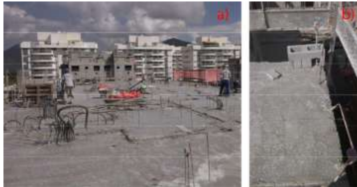
Figure 4. a) Image of grout points and b) iron axes placed before concreting to indicate the marking and location of the blocks.
