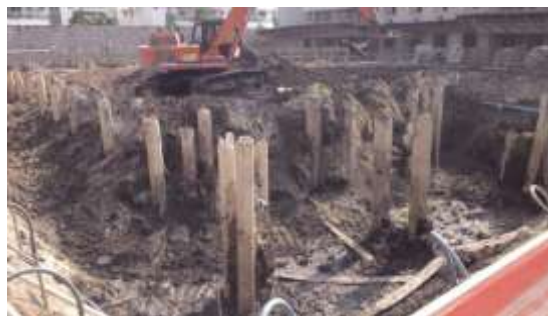
Figure 1. Foundation using precast concrete stakes.
