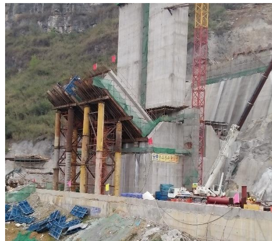
Figure 4 On-site construction image of the scaffolding
