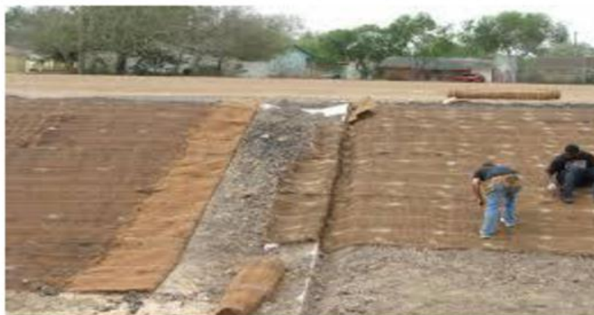
Figure 2: Blanketing technique
