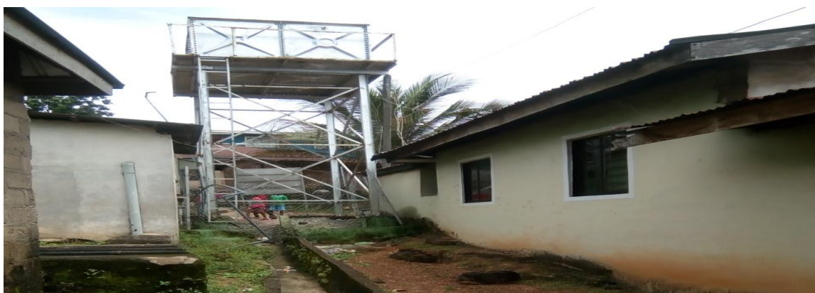
Figure 1 Household drinking water borehole sited in close proximity with the gutter and septic tank in the study area (both buildings have septic tanks by their sides), wellhead is directly under the overhead tank.
