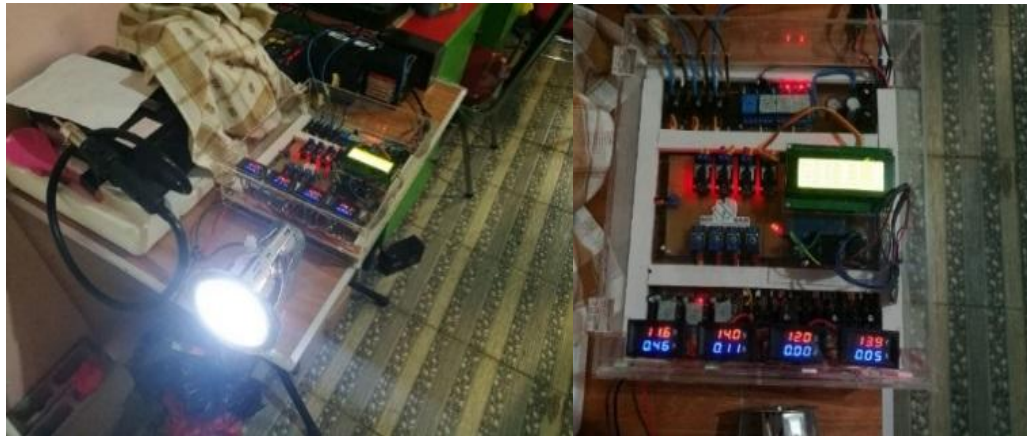
Figure 5 Prototype 3 battery power supply
