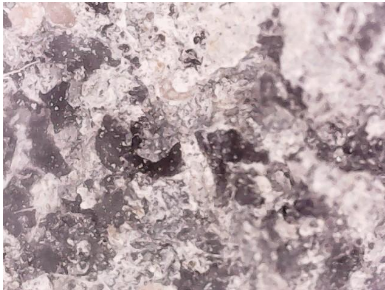
Fig.10: Rubber Concrete Failure Surface with Radiation at Microscope Level
