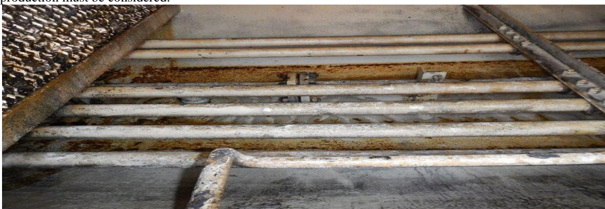
Figure 5: Vessel after cleaning
