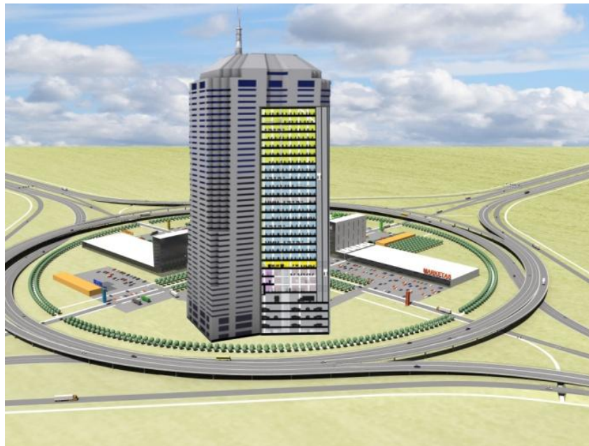
Figure 4: PINAVIA junction with an internal infrastructure
