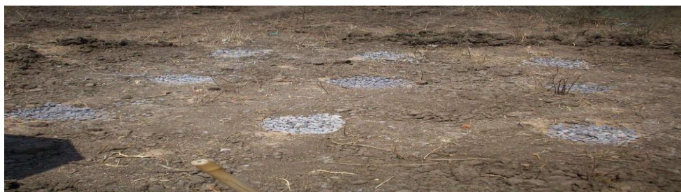
Fig. 1 Installed Granular piles below the flooring panel
