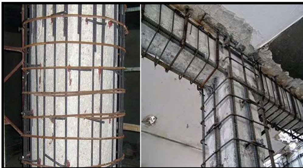
Figure 1.2: Strengthening of concrete elements
