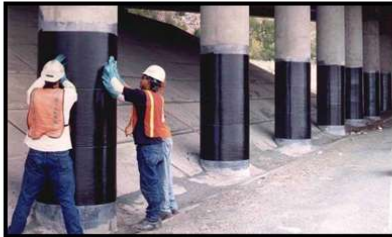
Figure 1.7(e): Strengthening with FRP
