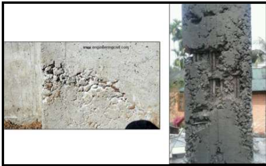
Figure 1.6: Nested column's concrete
