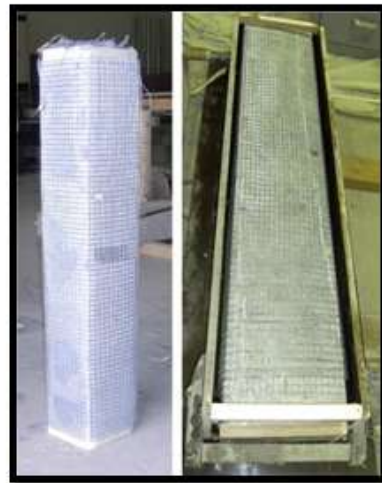
Figure 1.7(b): Ferro-cement jacketing
