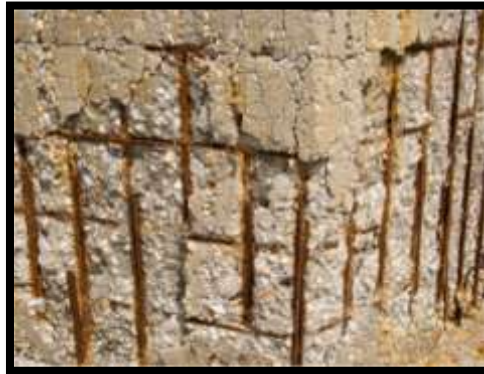
Figure 1.3: Rusty reinforcement and falling of concrete cover
