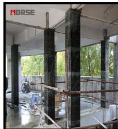
Figure 1.7(d): strengthening with carbon sheets
