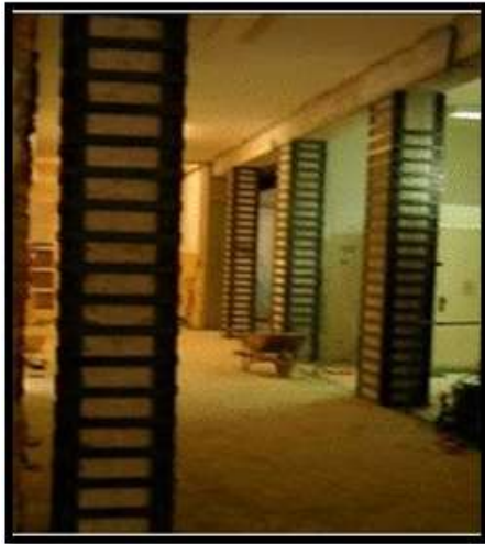
Figure 1.7(a): steel plate jacketing
