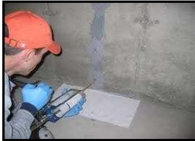
Figure 1.1: Concrete crack repairing with epoxy injection
