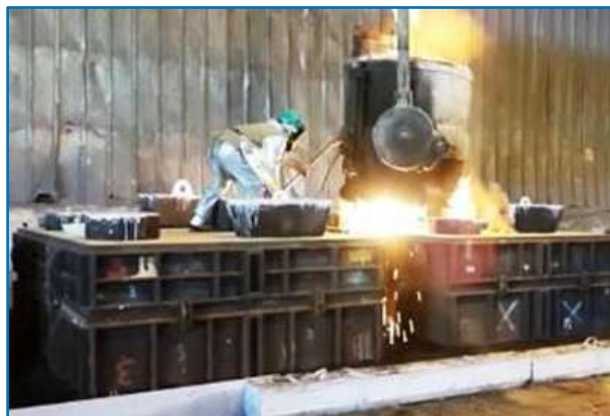
Figure 9: There are almost no emissions, exhalations during pouring.
