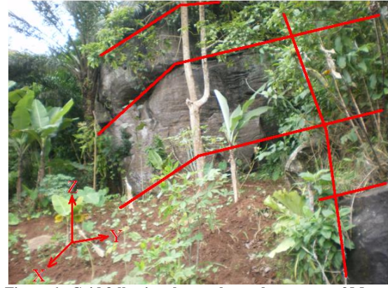
Figure 6 : Grid following the cracks on the outcrop of Mvog-Betsi (N03°51'49,8'' ; E11°28'27,5'' ; H = 861 m) [25]
