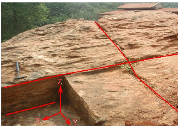
Figure 7 : Grid following the cracks on the outcrop of Nkolbisson (N03°52'06,8'' ; E11°27'28,5'' ; H = 733 m) [25]
