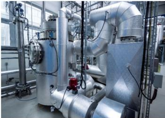
Fig. 2 LOCA Laboratory (Left – Gas separator, Center – H2 simulation vessel)
