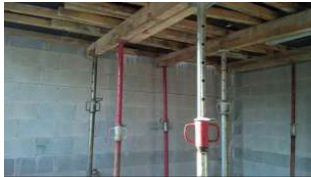
Figure 2. Image of the forms used in a structural masonry construction.
