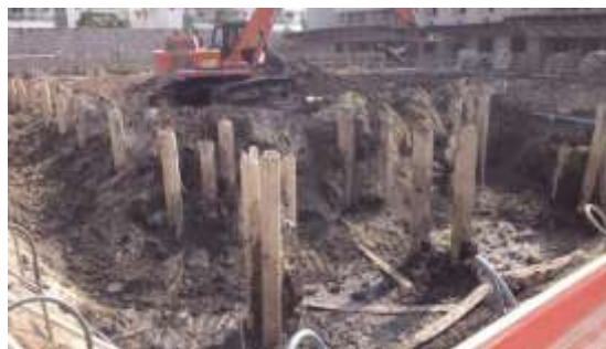
Figure 1. Foundation using precast concrete stakes.
