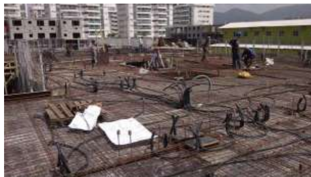
Figure 3. Image of the execution of the negative and positive frames as well as the electrical installation in the slab.
