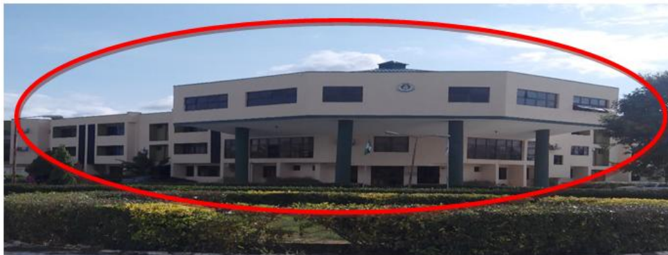
Exposed Council Chamber at Southern Side without adequate vegetations/trees
