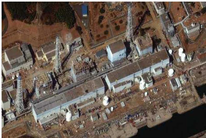
Fig.4The damaged reactor buildings at Fukushima Daiichi (Photo: Reuters/DigitalGlobe/Handout
