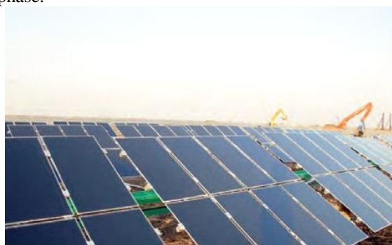
Fig. 6 Solar power plant
