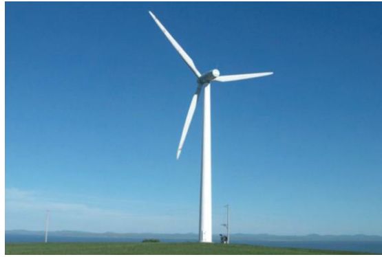
Fig. 3 Horizontal axis wind turbine
