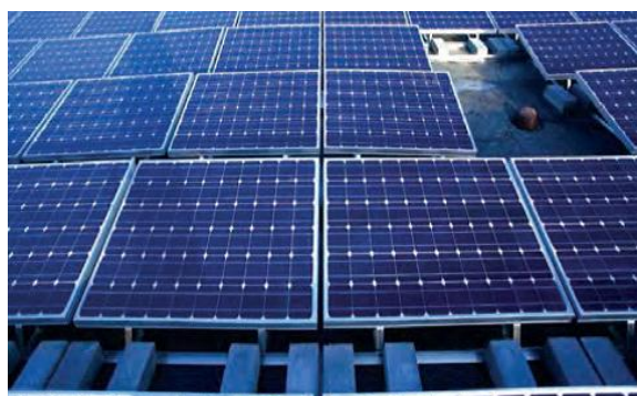
Fig. 7 Solar power plant
